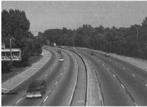
Figure 3 Level of Service A
