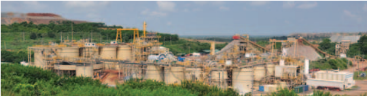
Chatree plant with the recently completed expansion plant
