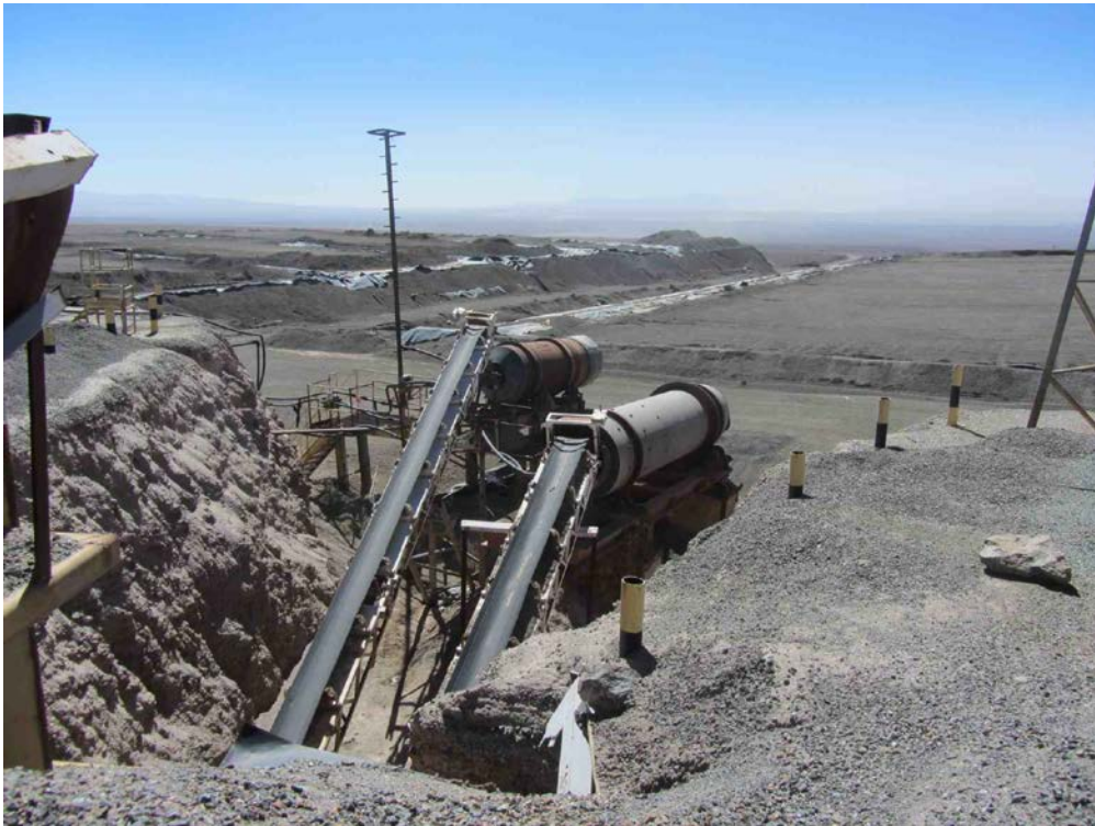
Figure 3 An abandoned copper oxide plant at Tuina
