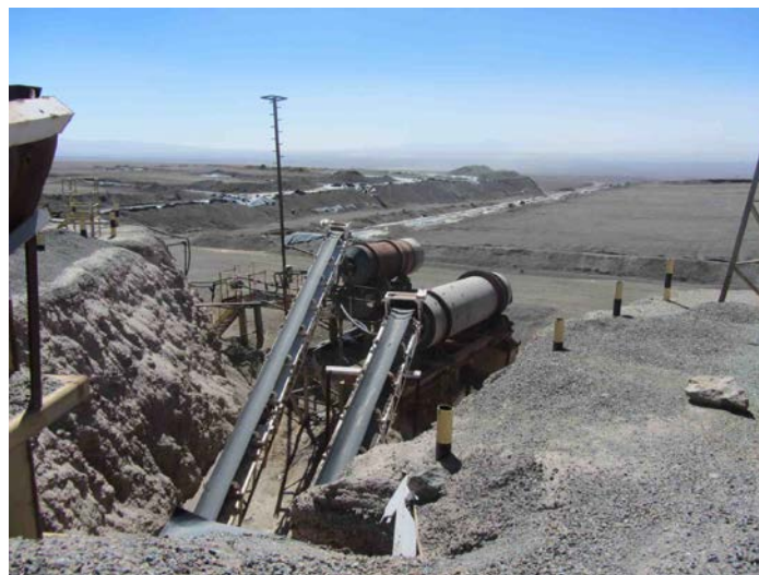
Figure 6 An abandoned copper oxide plant at Tuina
