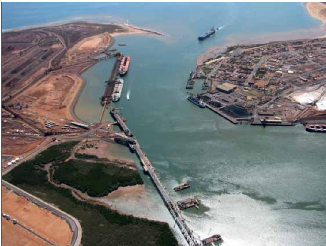
Figure 2 – Port Hedland port
