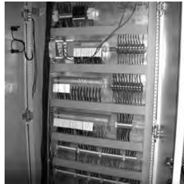
Figure 3: PLC, equipment-control substation, and communication interface
