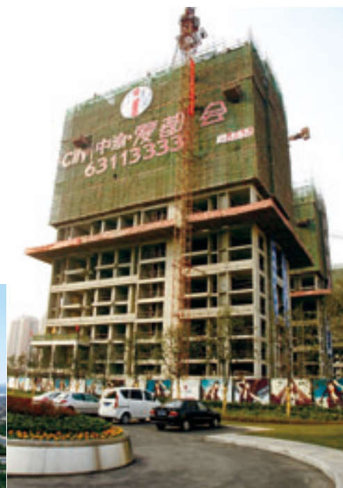
Construction Site of i-City
