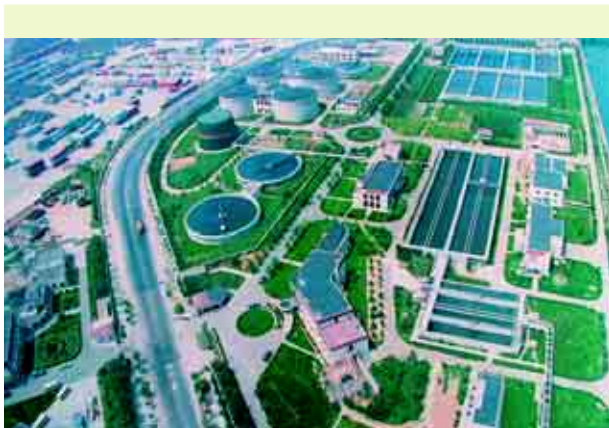
青島海泊河污水處理廠 Qingdao Haibohe waste water treatment plant
