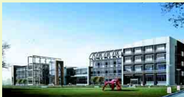
蘇能垃圾焚燒發電廠－生活樓 SuNeng waste-to-energy plant – Dormitory building
