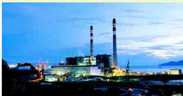
媽灣電廠 Mawan Power Plant
