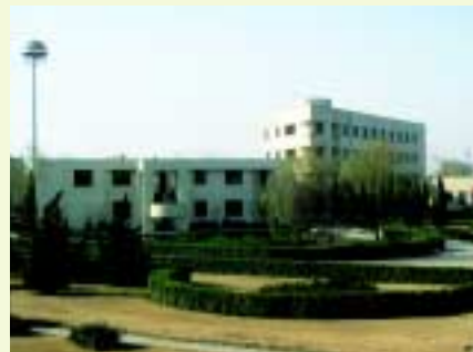
Zibo Waste Water Treatment Plant (Office building) 淄博污水處理廠（辦公樓）
