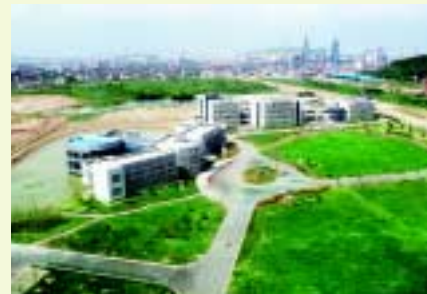
Suzhou Waste-to-energy Plant (Dormitory building) 蘇州垃圾焚燒發電廠（生活樓）
