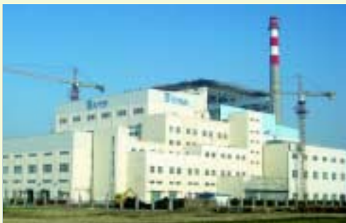
Yixing Waste-to-energy Plant 宜興垃圾焚燒發電廠
