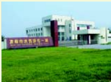
Jinan No. 1 Waste Water Treatment Plant 濟南市水質淨化一廠
