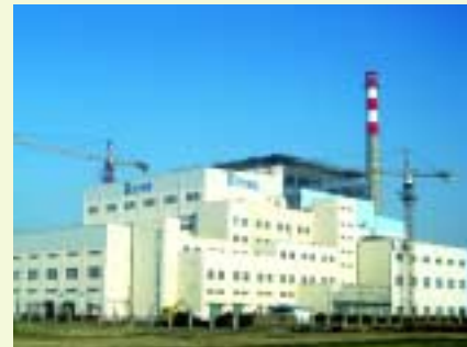
Yixing Waste-to-energy Plant 宜興垃圾焚燒發電廠
