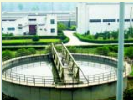
Zibo Waste Water Treatment Plant 淄博污水處理廠
