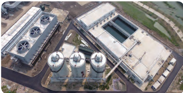
Leachate treatment system 成套滲濾液處理系統
