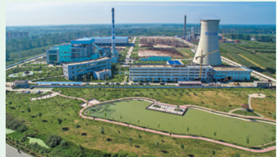
Dangshan Integrated Biomass and Waste-to-energy Project 礪山生物質及垃圾發電一體化項目
