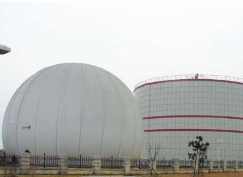
digester and methane storage tank of Maidaowaste Water Treatment Plant 麥島污水處理廠消化池與沼氣罐
