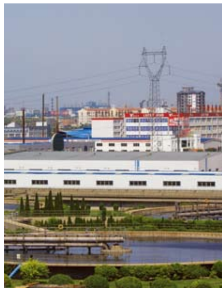
Zibo Waste Water Treatment Plant 淄博污水處理廠
