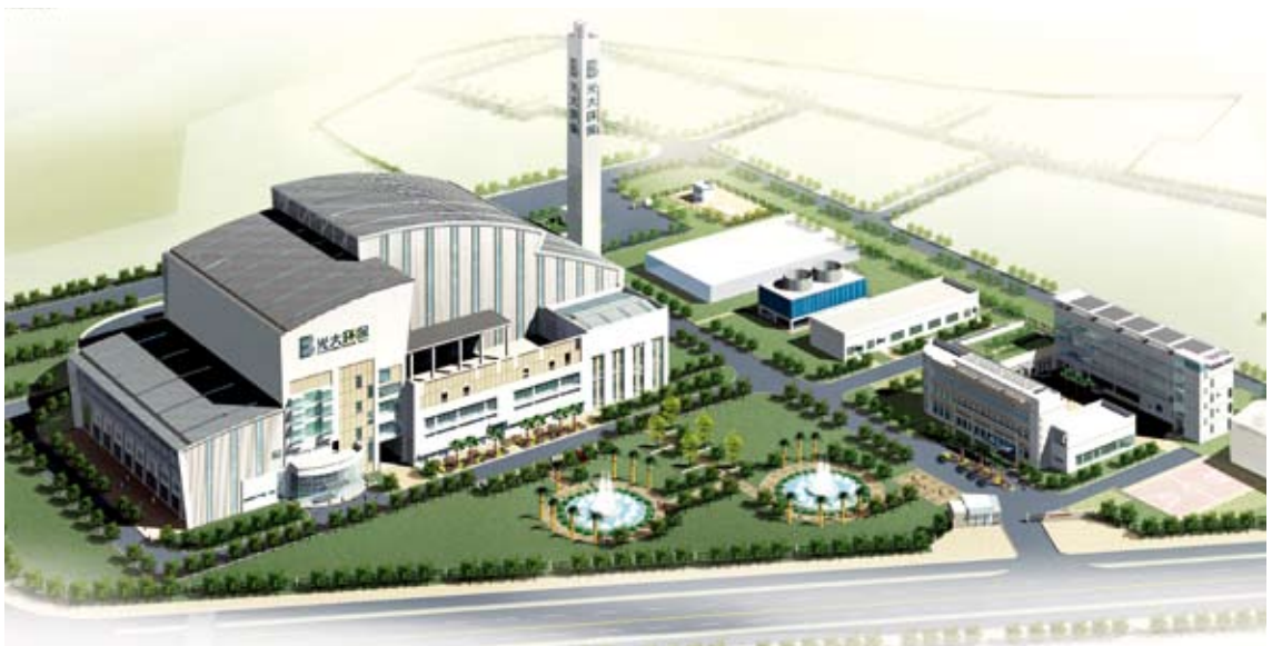
Changzhou Waste-to-energy Plant 常州垃圾焚燒發電廠
