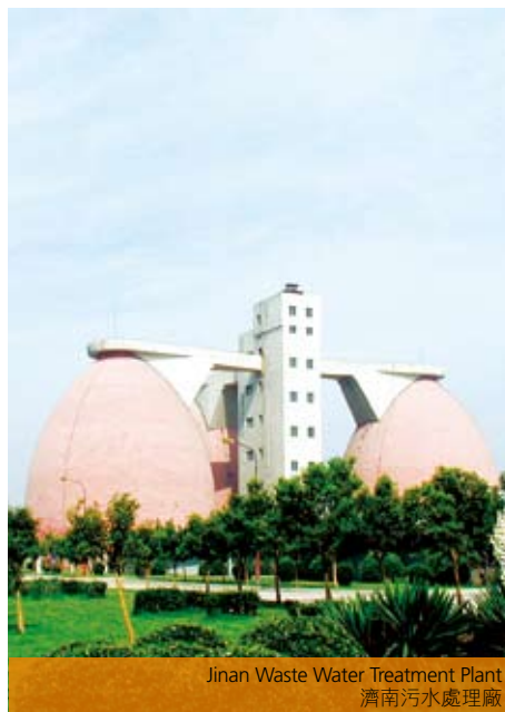
Jinan Waste Water Treatment Plant 濟南污水處理廠
