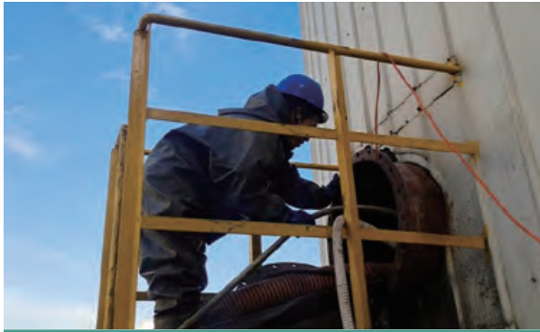
Shandong Linshu waste-to-energy project conducted equipment maintenance and safety inspection rectification actions 山東臨沭垃圾發電項目開展設備檢修及安全隱患排查整治行動
