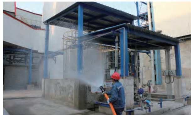
Jiangsu Rugao biomass direct combustion project conducted an emergency drill on ammonia leakage 江蘇如皋生物質直燃項目開展氨水洩漏事故應急救援演練
