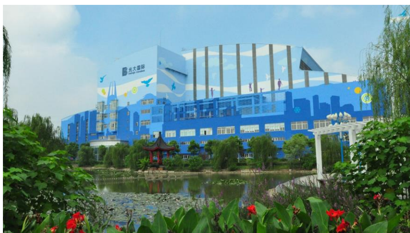
Jiangsu Changzhou Household Waste-to-energy Project
