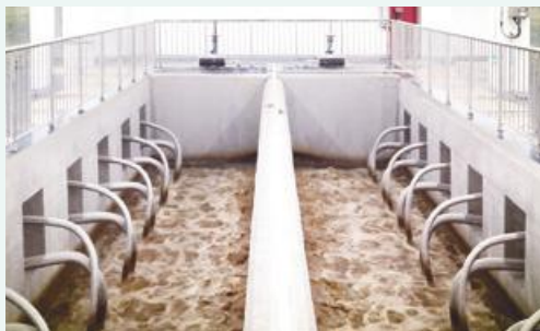
Ji'nan Huashan Waste Water Treatment Project 濟南華山水質淨化項目
