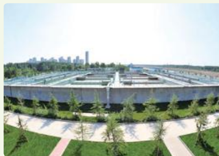
Ji'nan Waste Water Treatment Project
