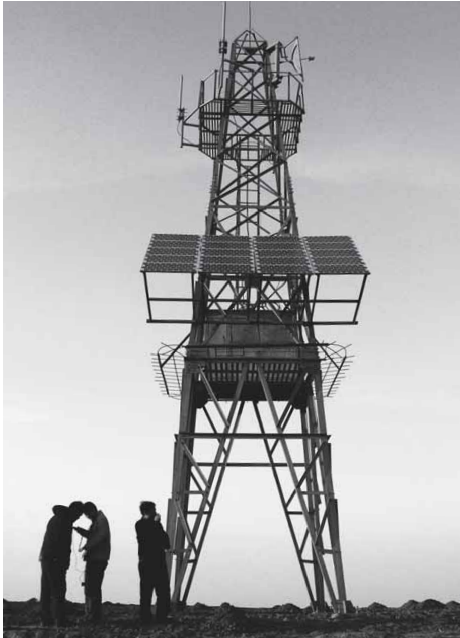
Telecommunications Infrastructure Project
