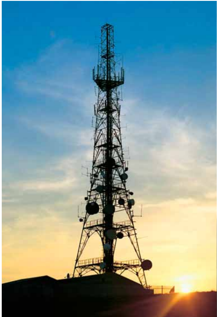
Base Station Maintenance Projects
