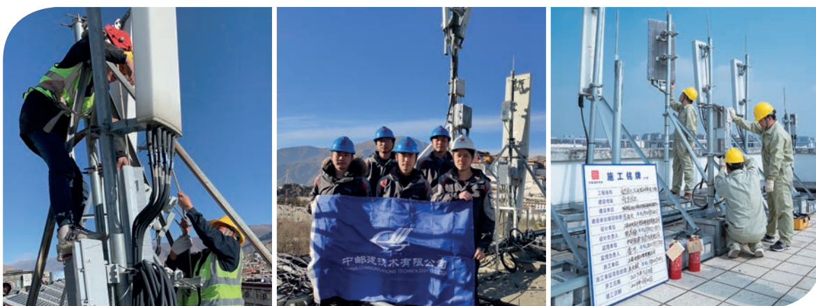
The Group undertook 5G base stations construction
