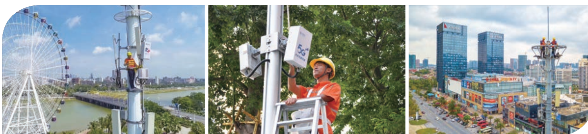
The Group supported domestic telecommunications operators in 5G construction
