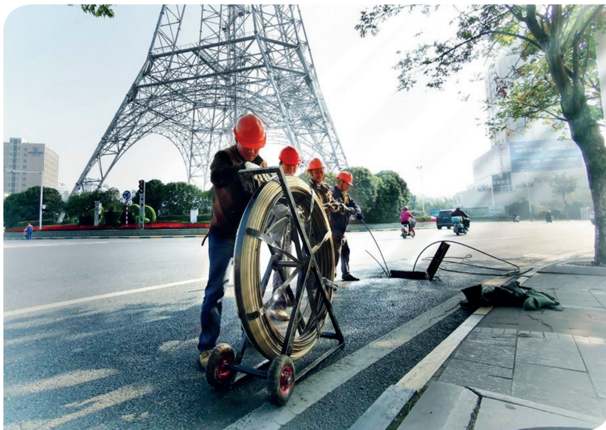
The Group undertook communications network construction project
