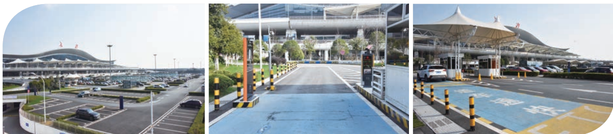
The Group provided Smart Parking (ETC system) integrated solution for airport
