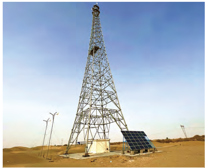
Building solar energy base station in Xinjiang.
