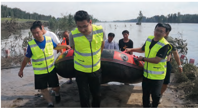
Emergency Communication Cable Repair Across the Juma River in North Baoding, Hebei.
