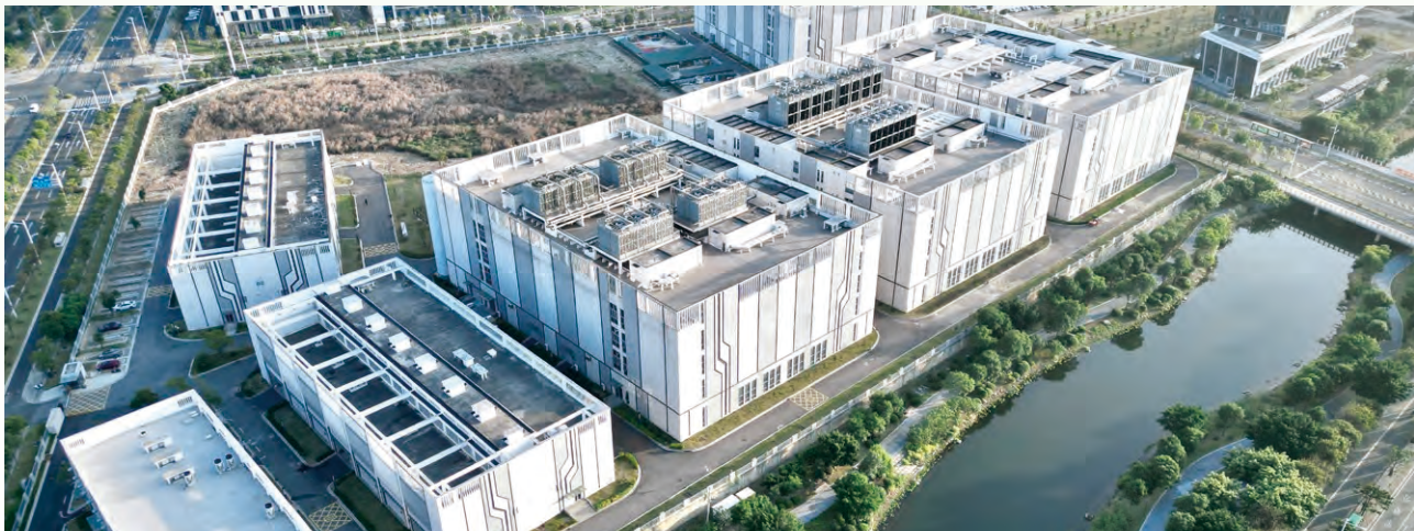
China Mobile (Fuzhou, Fujian) region level ultra-large data center.
