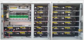
The echelon use of traction batteries
