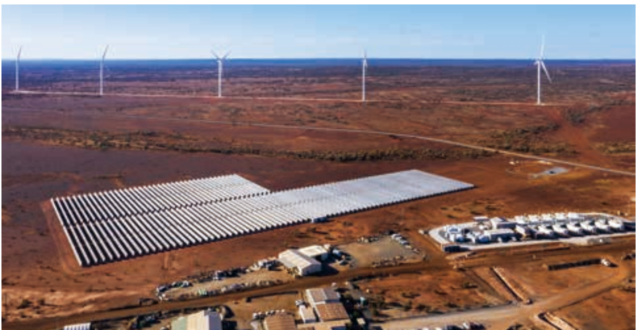
EDL's Agnew Hybrid Renewable Microgrid 56MW is first in the country to utilise wind generation on a large scale at a mine site
