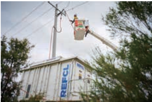
Powercor installation of Rapid Earth Fault Current Limiters
