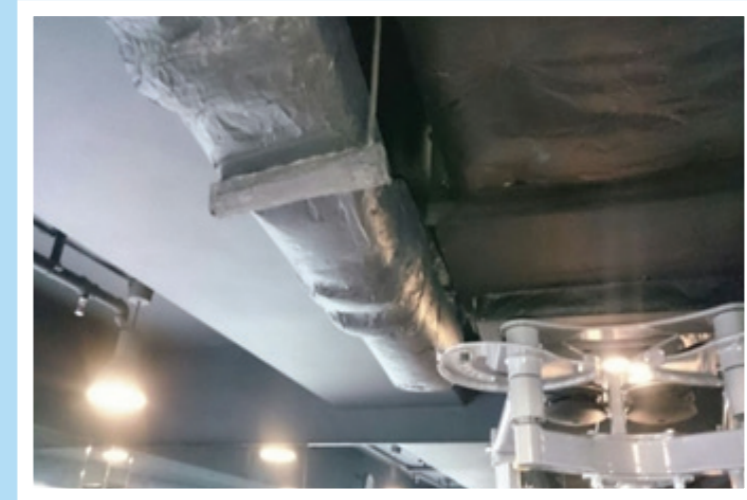
Use anti-collision material to wrap the shroud bracket
