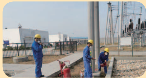
Emergency drill on transformer fire of Wuhe Yinmahu Wind Power Project 五河飲馬湖風電場現場變壓器著火應急演練
