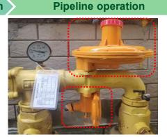
Replace old regulator by parts to avoid overall replacement and reduce operating costs
