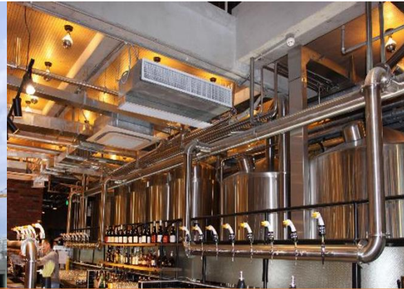
Craft beer technology, equipment, system and engineering
