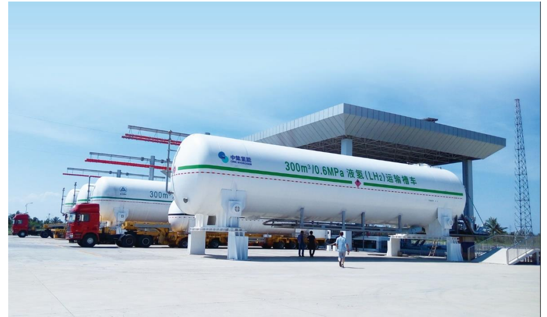
High-vacuum multi-layer winding adiabatic liquid hydrogen storage tanks in Wenchang Satellite Launch Base in Hainan, with the capacity of 300m 3 and the work pressure of 0.6MPa
