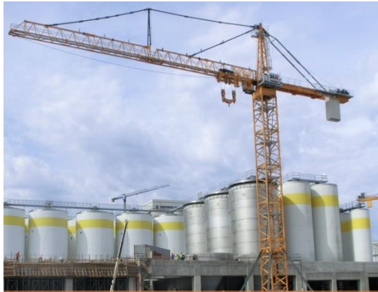
Large brewery fermentation tank and project
