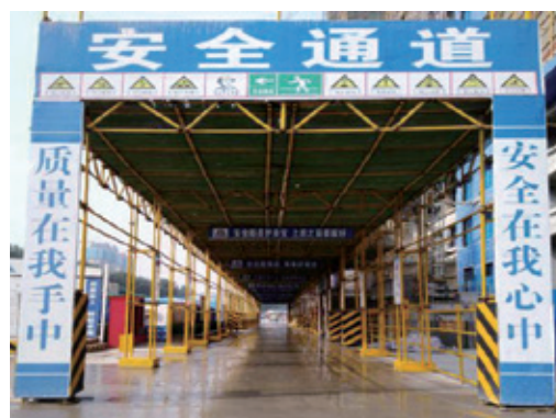
Figure 7: Major safety passage at a construction site
