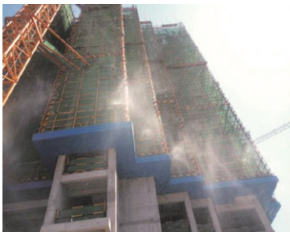
Figure 9: External sprinkler system at construction site Figure 10: Solar street lights at construction site
