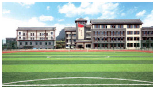
Figure 18: Primary school constructed under the assistance of the Group
