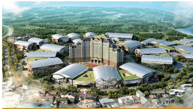
The total area of roof PV system is 58,000 m 2 and the annual electric energy production reaches 8 million kWh.
