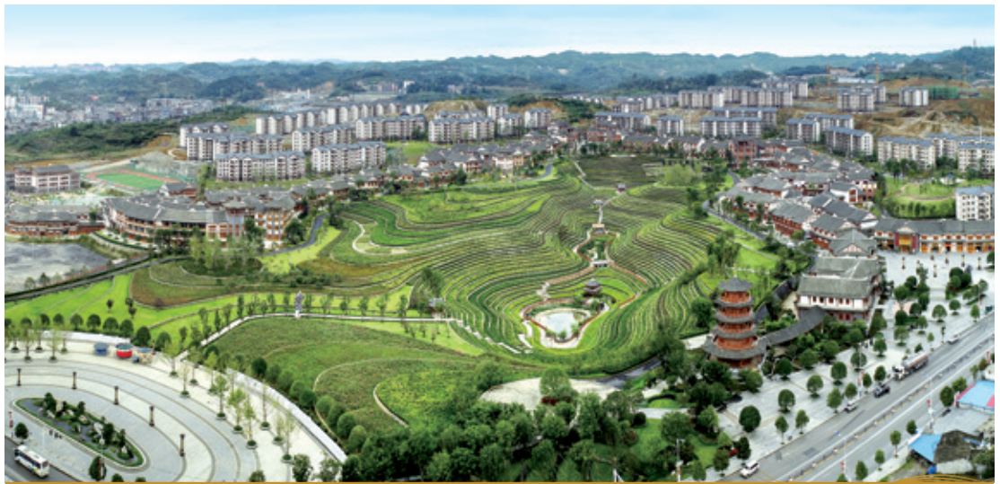
Relocation community for immigrant constructed under the assistance of Evergrande in its partner assistance with Bijie City — Shexiang Old Town
