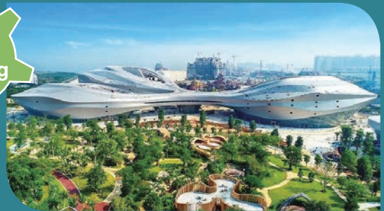
Integrated solar PV building
