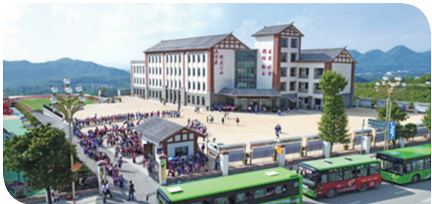
The Second Primary School of Evergrande constructed under assistance of the Group
