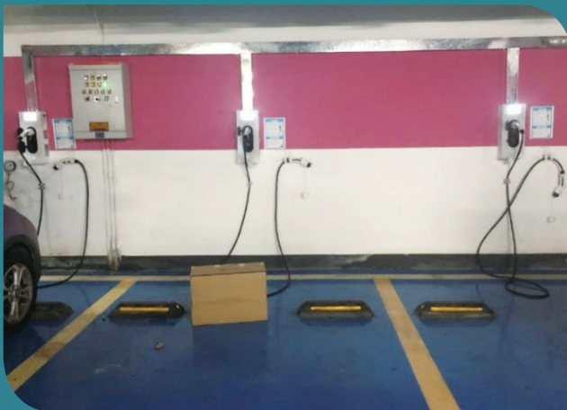
Installation of charging piles
