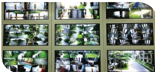
Fire Control Center
