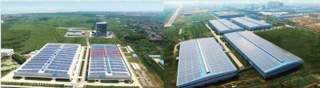
Overhead view of solar photovoltaic power generation system
