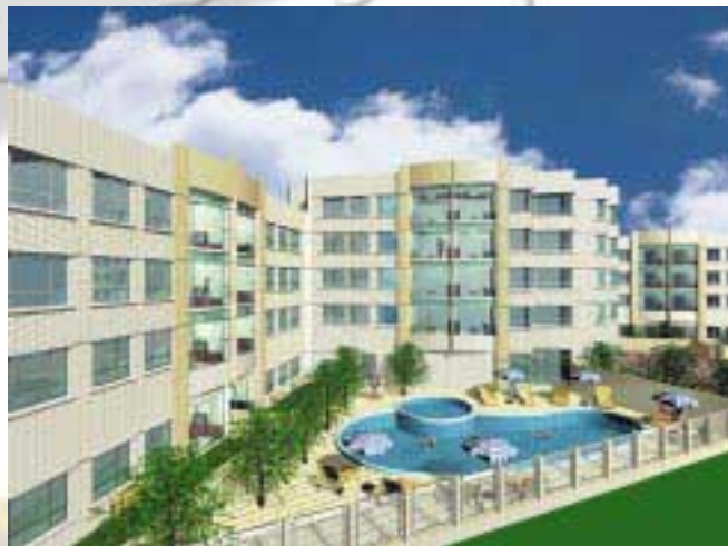
Low-density Residential Development at Tan Kwai Tsuen, Yuen Long 低密度住宅發展於元朗丹桂村
