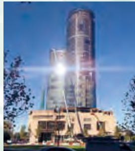
珀斯The Towers at Elizabeth Quay第9期竣工
