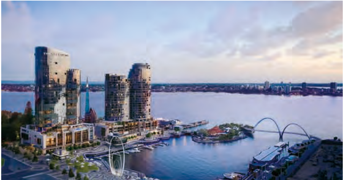
珀斯The Towers at Elizabeth Quay
