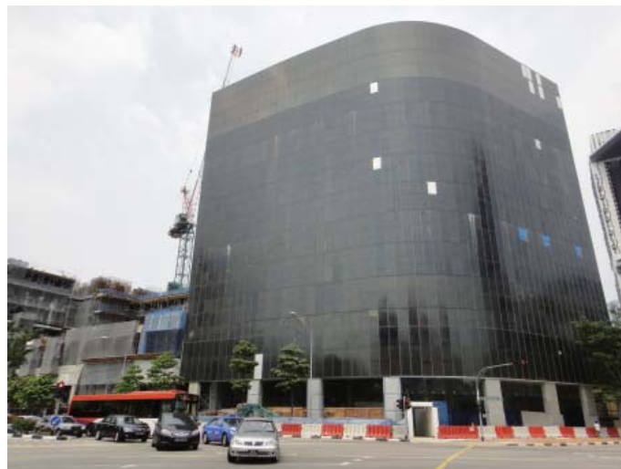
New Bridge Road/Outram Road/ Cantonment Road 交叉路口的面貌
