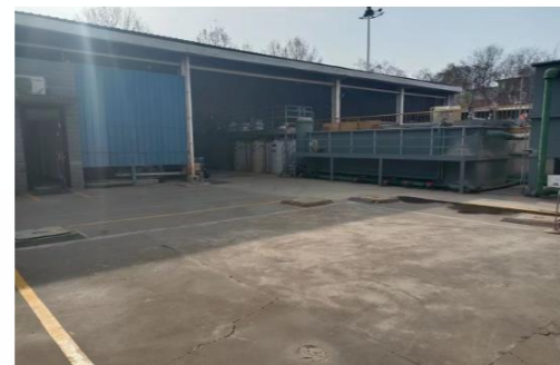
Industrial Wastewater Treatment Station
