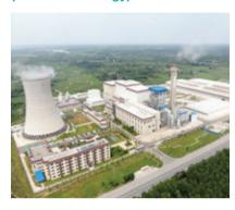
Built on a site area of 215 mu. Phase I of the household waste-to-energy project equipped with a mechanical grate furnace and a condensing turbine generator unit with a designed daily waste processing capacity of 400 MT and annual designed on-grid power generation volume of 47 million KWh to realise the reduction, recycling and detoxification of household waste and convert waste into value.
