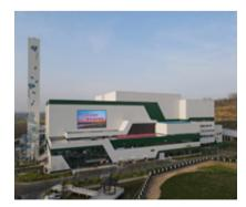
Located at the west side of Xiaomopan Hill in Liuhe District, Nanjing, the project offers a daily household waste processing capacity of 1,000 MT and an ash landfill with a capacity of approximately 350,000 cubic metres. Fume purification process technologies adopted include in-boiler  $\text{deNO}_{\text{x}}$ , ex-boiler catalytic reduction  $\text{deNo}_{\text{x}}$ , semi-dry deacidification, active carbon spray, dry-spray deacidification and dust removal bag.
