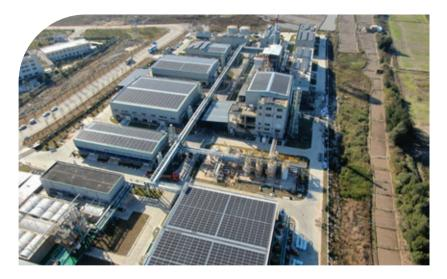
Wenling Solid Waste Treatment Project has constructed solar energy facilities at locations such as rooftops of the plant buildings, accident pools, preliminary rainwater captures with an installed area of approximately 12,000 m², and an aggregate installed capacity of approximately 1.6MW.
