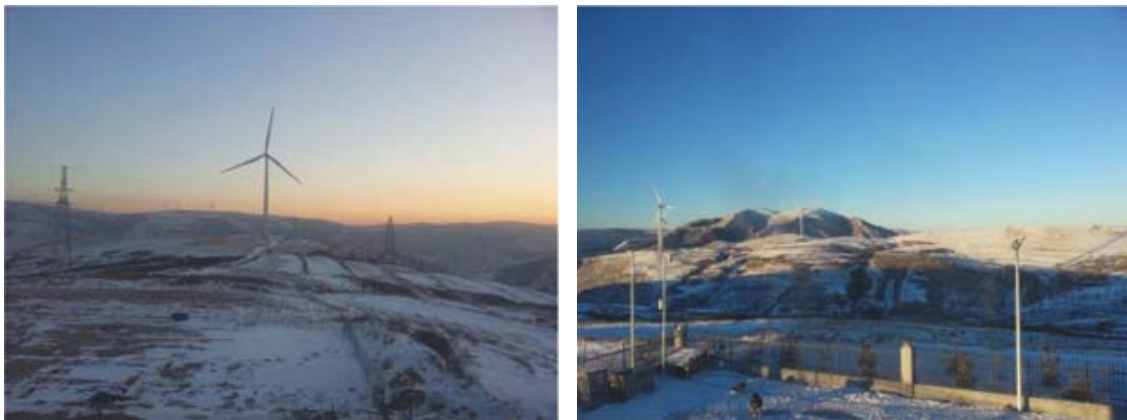
Figure 7.1 Ningwu Wind Turbine Generators
