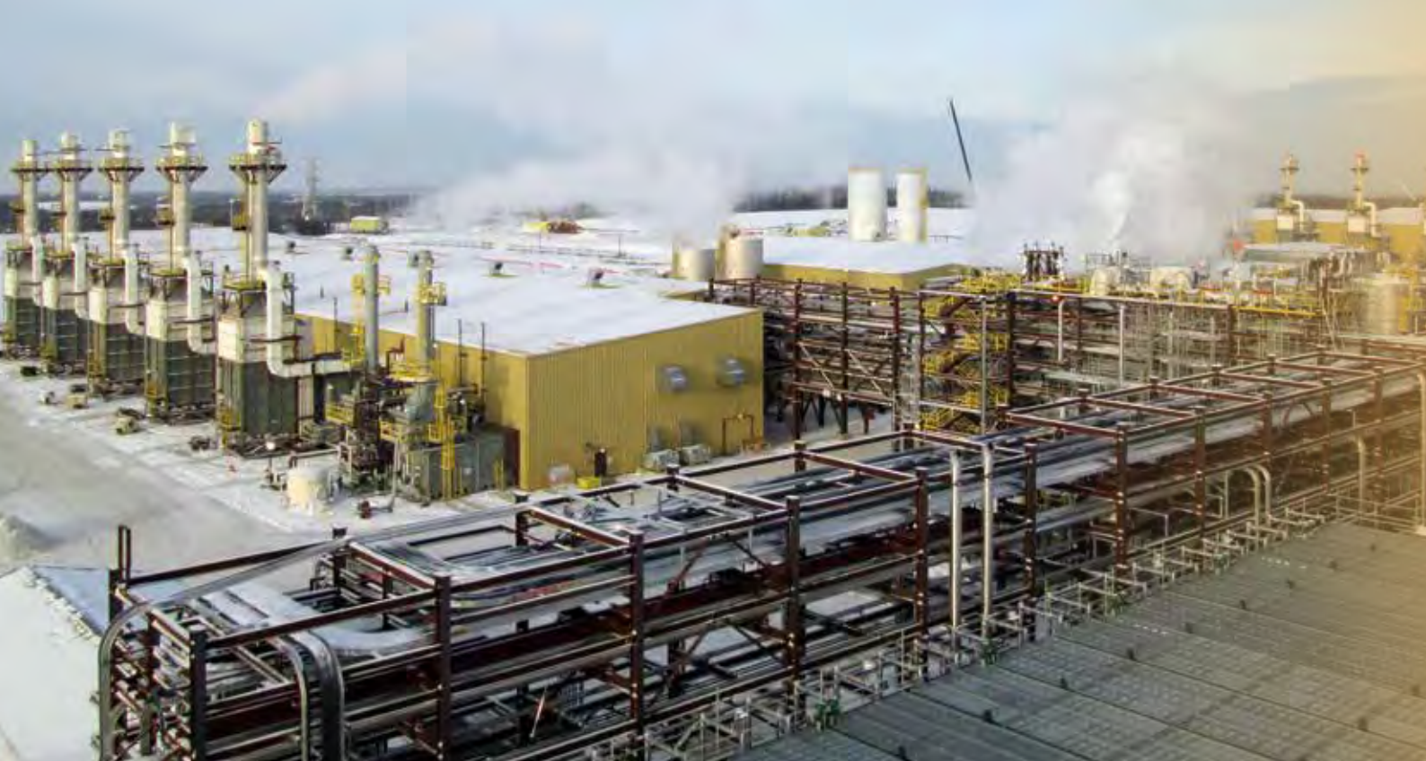
The Sunrise Energy Project commences steam operations.
