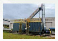
Two-stage activated carbon adsorption treatment equipment
