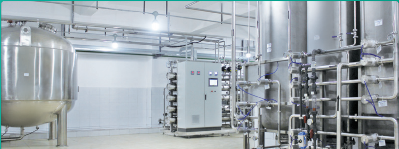
重慶康樂製藥有限公司（「重慶康樂」）— 廠區純化水系統 Chongqing Kangle Pharmaceutical Co., Ltd.* (“Chongqing Kangle”) — Water purifying system in the plant
