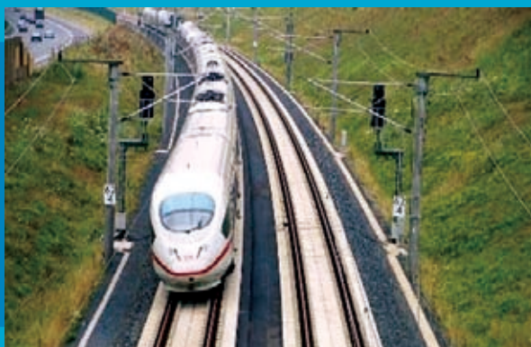
用「泰立」水泥建成的京滬鐵路莊段 The Zaozhuang section of the Beijing-Shanghai Railway, made of cement under the brand "Titan"
