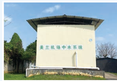
Reclaimed water reuse system 中水回用
