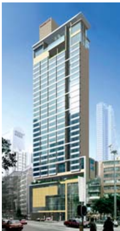
Leighton Road project
