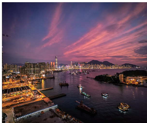
NKIL 6549, West Kowloon Waterfront Residential Development, Hong Kong
