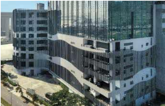
Vehicular ramp access to every warehouse floor
