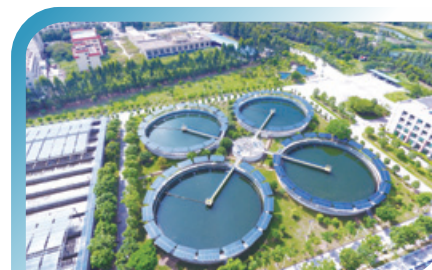
Distributed Photovoltaic Power Station in a water plant of BEWG, Dongguan, Guangdong Province
