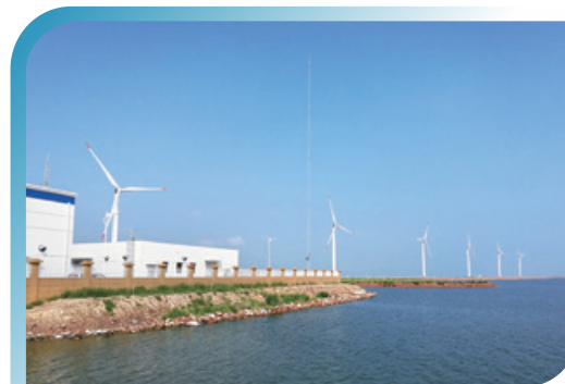
Centralised Wind Power Plant, Binzhou, Shandong Province
