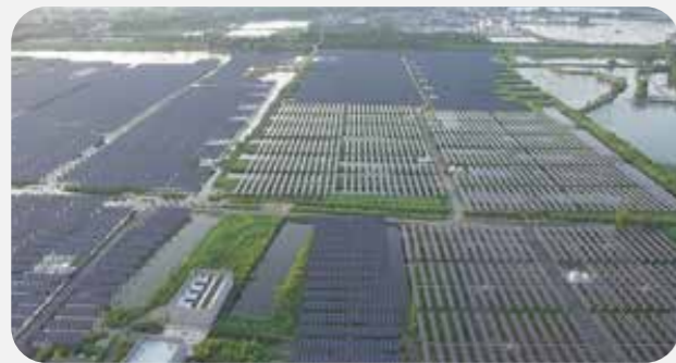
Centralised Photovoltaic Power Plant, Weishan County, Shandong Province 山東省微山縣集中式光伏發電站
