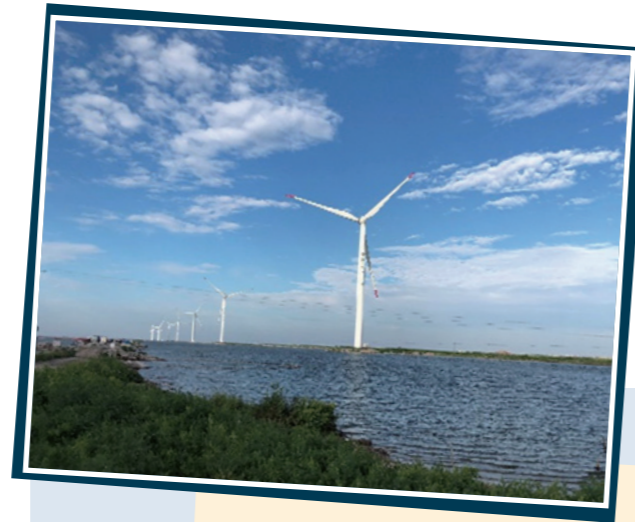
Lusa wind power plant in Shandong Province
