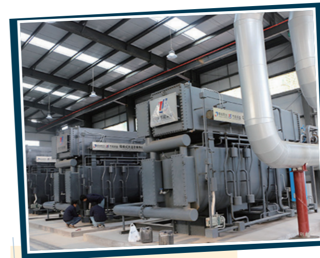
Yongheng clean heat supply project in Ningxia
