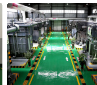
Channels for inspection
