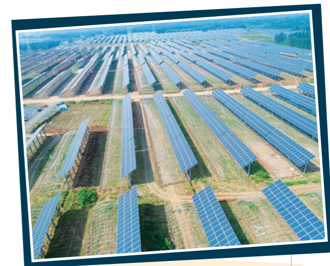
Centralised photovoltaic power plant in Xintai City, Shandong Province
