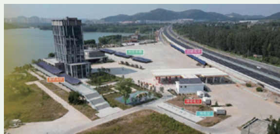
Integrated smart energy project in Jinan (Gushan) Service Area of the Beijing-Taipei Expressway
