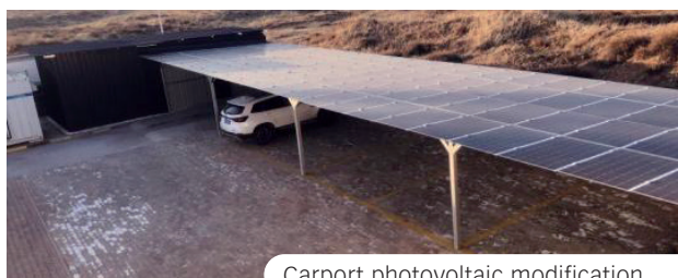
Carport photovoltaic modification
