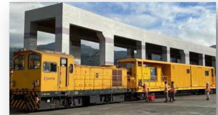
Train Maintenance Containers
