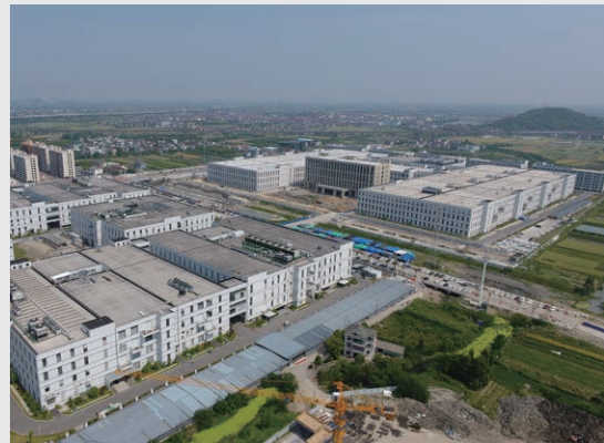
| Road Improvement in the Yuyao Chengxi Production Base
