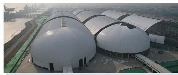
Closed Greenhouses at Jingjiang Port
